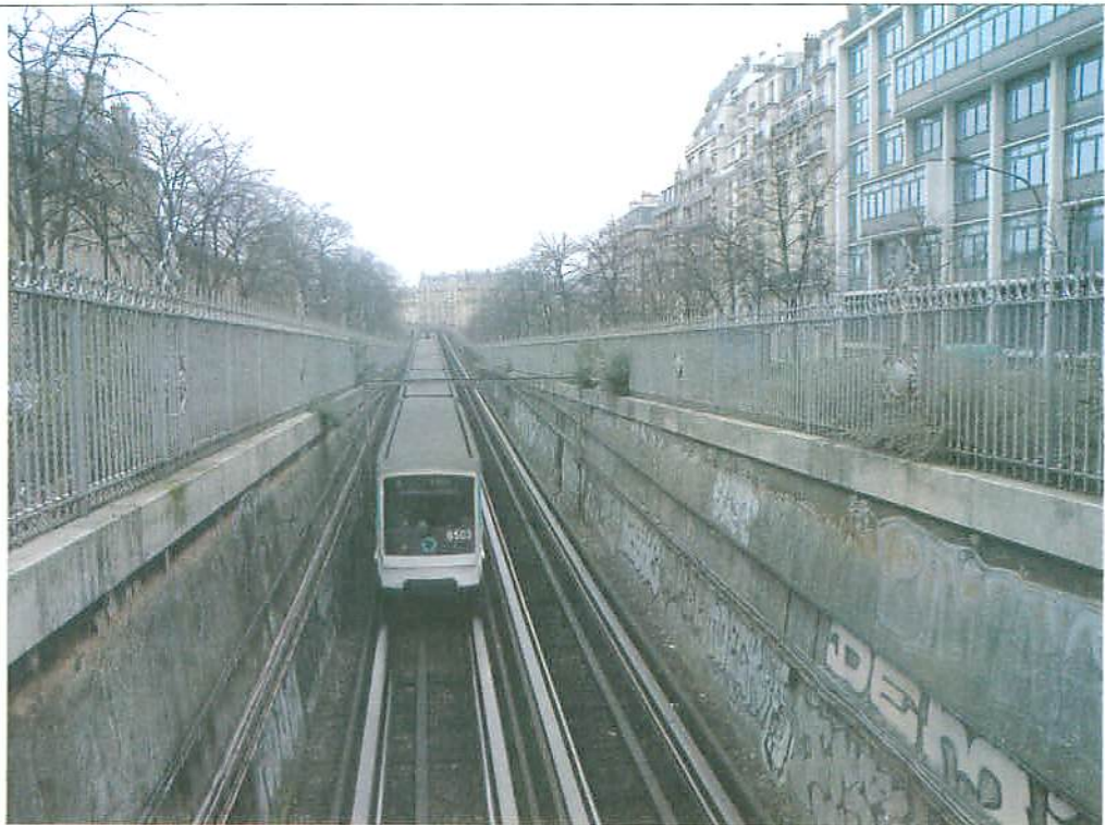
Surface lines may cause vibration or vibration-induced noise
